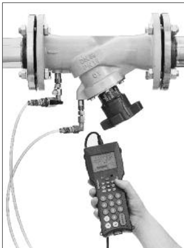
Flow-meter "OV-DMC 2", item no. 106 91 77 with "Hydrocontrol F/FR/FS"
