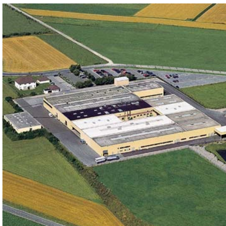
Production facility in Brilon
